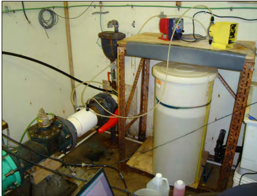
Photo 5. Automated water quality monitoring apparatus in CBWS chlorination shed, operated by Ministry of Environment Water Stewardship. 17-Jul-07
