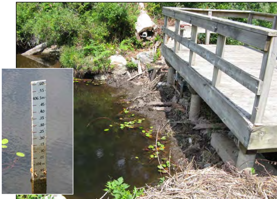
Photo 8. Grafton lake outlet dam during summer draw-down. Inset shows staff gauge indicating a water level of 104.87 m on that date. Note remote-control video camera in log on far side of dam, used to monitor beaver activity. 23-Jul-09
